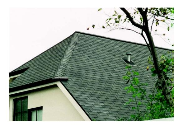
Asphalt shingle roofs provide a relatively low maintenance, corrosion-resistant roofing system. There are a number of specification and installation steps to follow to achieve maximum serviceability from these roofs. This bulletin outlines the design and installation criteria for achieving a successful asphalt shingle roof.
