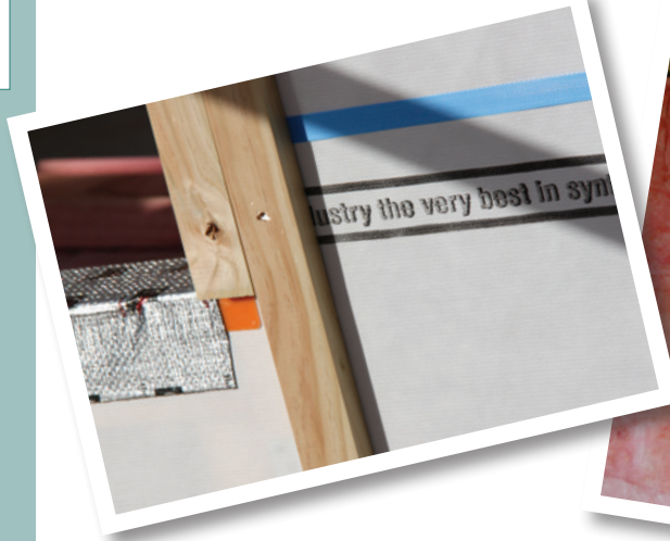
1 TIMBER CAVITY BATTEN INSTALLATION
