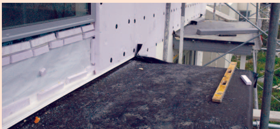
Gaps must be maintained between the bottom of the cladding and any roof surface or flashing below.
