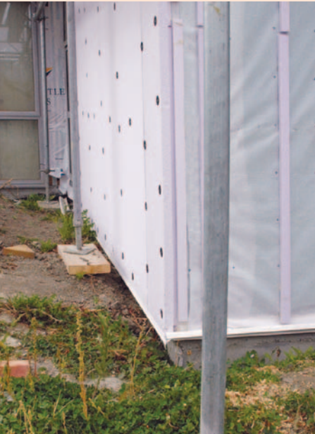
There are minimum clearance requirements between the bottom of the cladding and the adjacent natural ground or paving.
