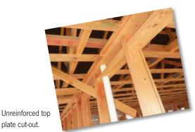
A large cut-out that the builder said would be repaired (but repairs are unlikely to be adequate due to the geometry). Appears to be a bracing wall re HD bolts.
