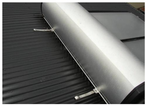
Stainless steel (like these solar water heater straps) should not be in direct contact with zinc/aluminium-coated roofing in exposure zone D or where exposed to salt spray.
