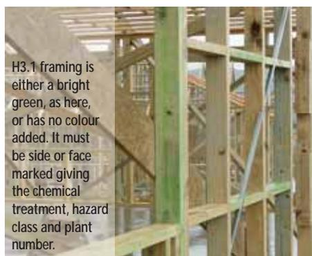
H3.1 framing is either a bright green, as here, or has no colour added. It must be side or face marked giving the chemical treatment, hazard class and plant number.
