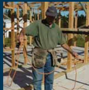
As you bring the loops together give the lead a slight twist between your thumb and forefinger. This will ensure each loop hangs straight.
