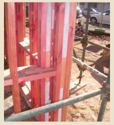
Figure 1: Insulation needs to be installed beforehand in all areas that cannot be accessed after the building wrap is installed. In this case, the insulation is grey.
