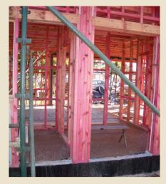
Figure 2: The stud to stud butt joint (thermal bridge) common on most sites today, where framing is constructed off-site.
