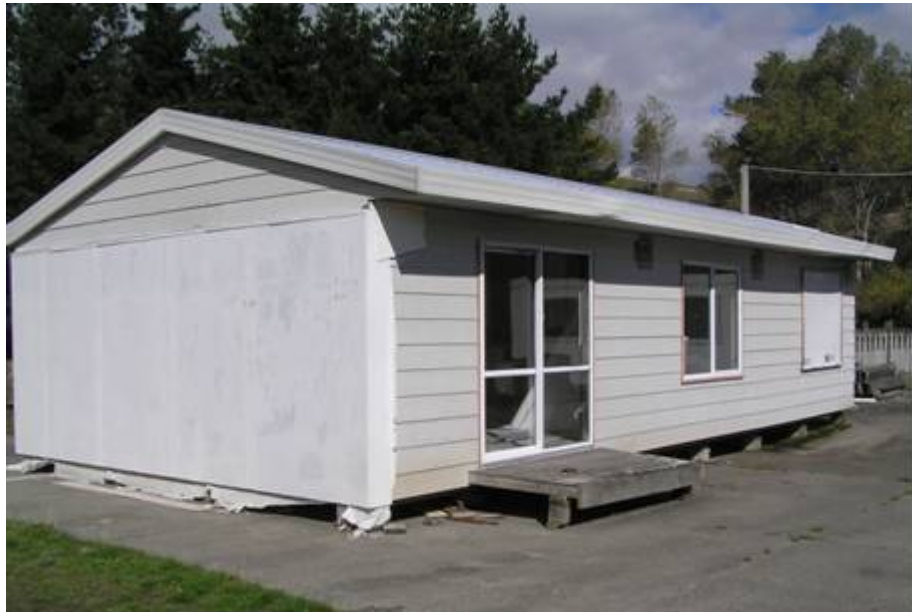
Figure 3: Fire test house – sprinkler pipework installed in roof space.
