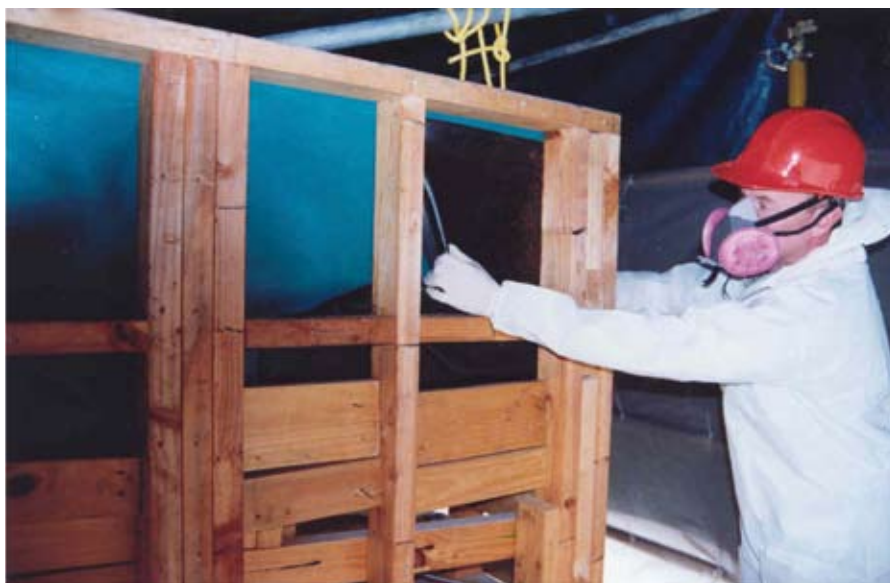
Carrying out an inspection in a contaminated environment.
