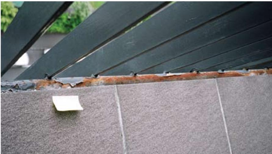
Poor specification and application of paint can result in corrosion that is very difficult to repair. Also, finishing the waterproofing onto the steel of the balustrade is unlikely to be successful.
