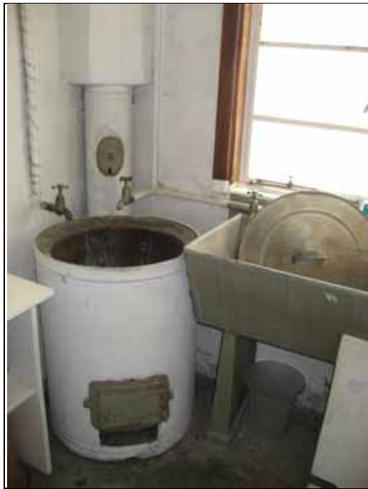
Figure 191: 1930s Laundry Copper
