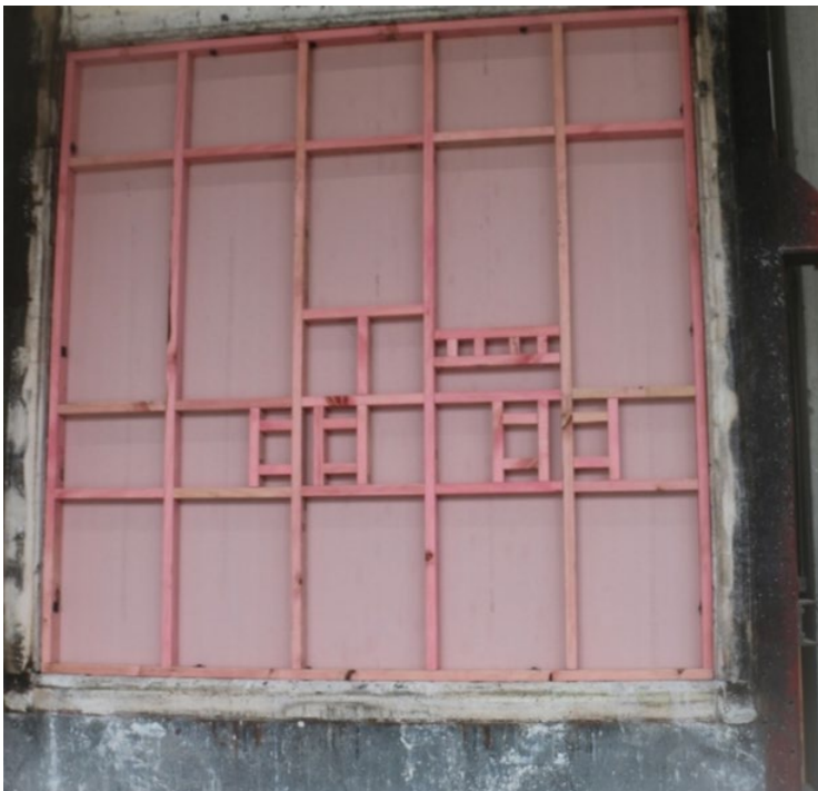
Figure 5. Plasterboard wall framing.
