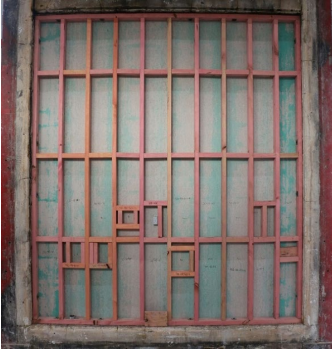
Figure 7. Fibre-cement board wall framing.
