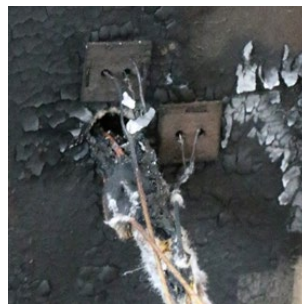
(c) Unexposed post-test
