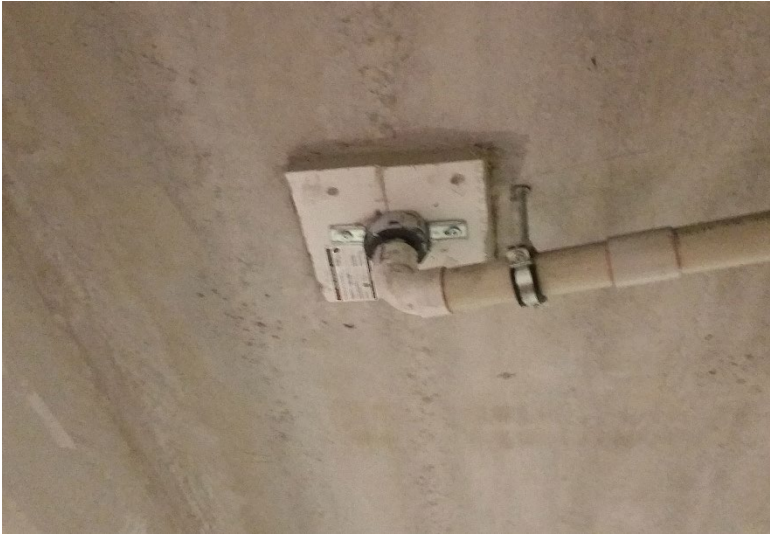
Figure 59. Plasterboard pattress covering a penetration through a concrete ceiling.
