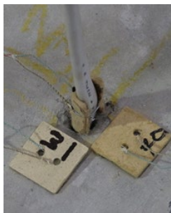
(b) Unexposed pre-test
