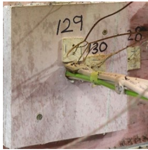
(c) Unexposed post-test
