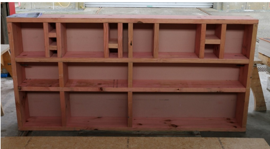
Figure 8. Plasterboard ceiling/strand board floor framing.
