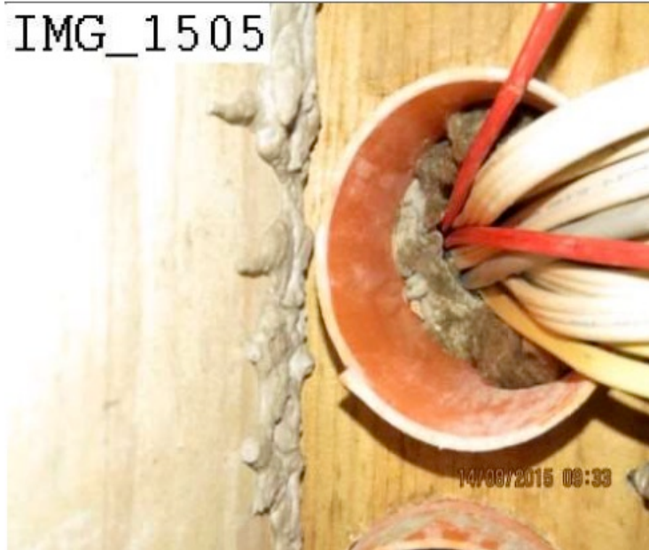
Figure 56. Cable bundle through timber infill floor.
